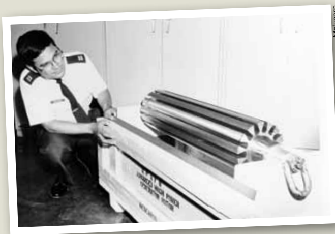
Officer measures Aero Propulsion Laboratory rotor for advanced high-energy alternator designed to produce up to 5 million watts of electricity
