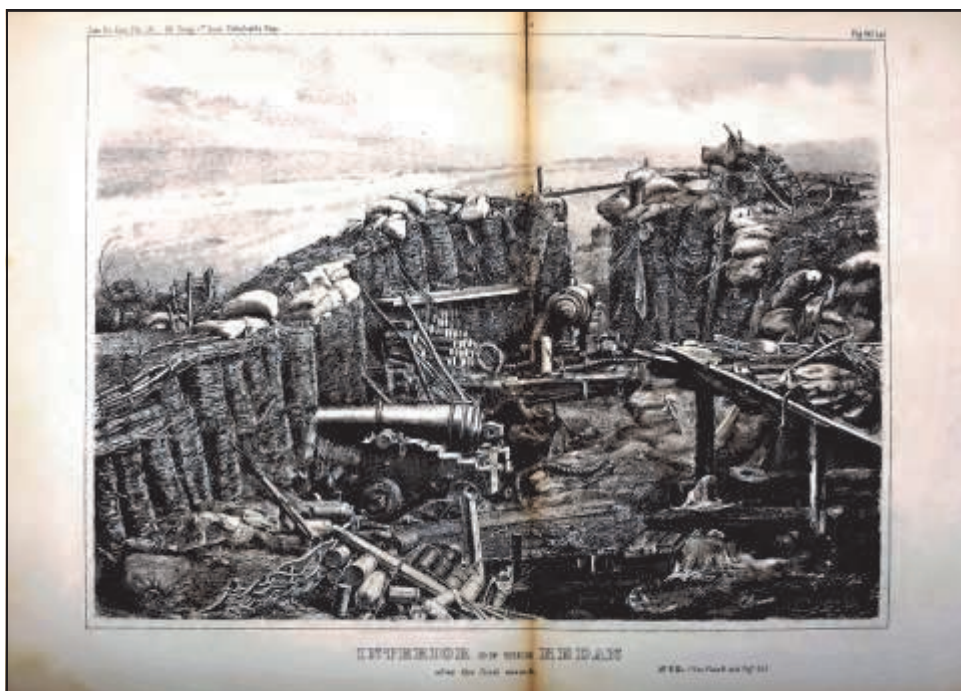
Post battle sketches of the Russian Fort Malakoff produced by the commission. They show masonry fortifications with the addition of field works as well as artillery positions within field works
