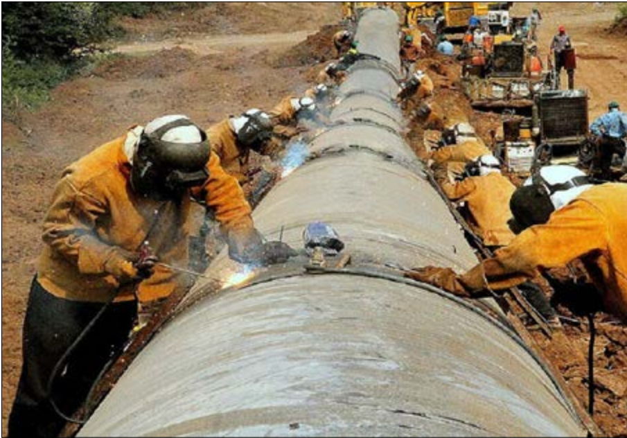
Workers construct a pipeline in Iran near Azerbaijan.
